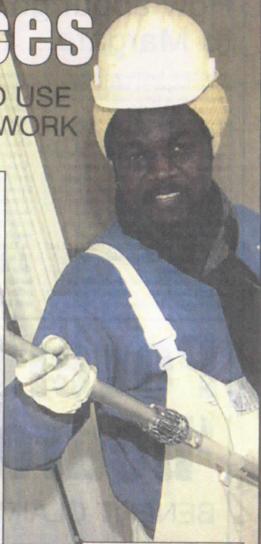
BRUSHING UP: Desi Mahusa helps paint a house in Brixton
